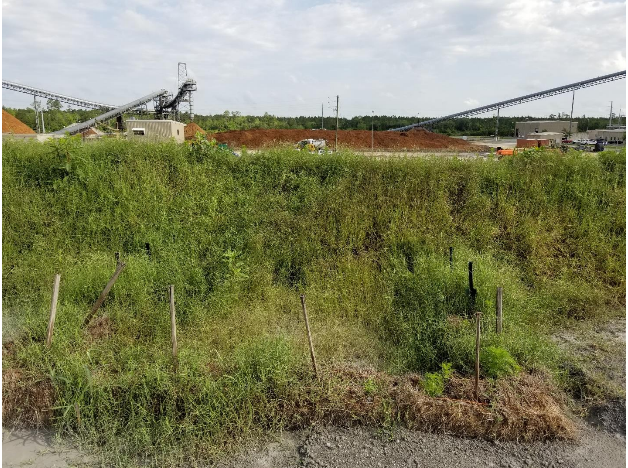
Figure C-1. Well-Established Vegetation Around Cell 2 Downcomer Inlet as Observed on 04/16/2020
