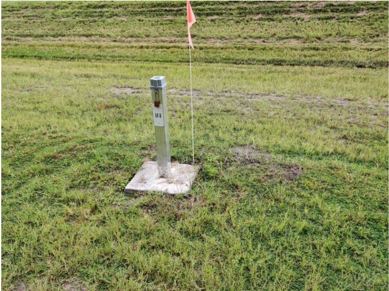
Figure C-5. Well-Maintained Vegetation around LF-3's Concrete Pad as Observed on 07/22/2020
