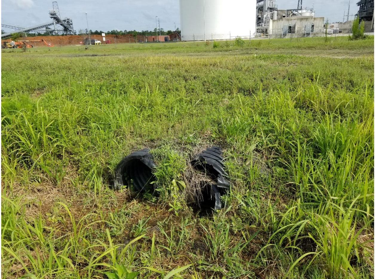
Figure C-3. Well-Maintained Vegetation Height around Cell 3 Culverts Inlet as Observed on 04/16/2020
