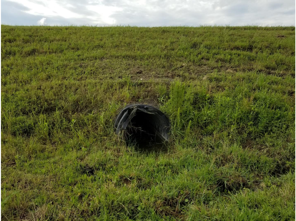
Figure C-2. Well-Maintained Vegetation Height around Cell 4 Culvert Outlet as Observed on 04/16/2020
